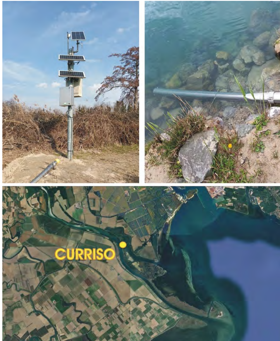
Figure 60 – Station CURRISO located in the Regional Nature Reserve of the Isonzo River Mouth. Automated remote station and the stilling pipe containing CTD instruments are also shown. I
