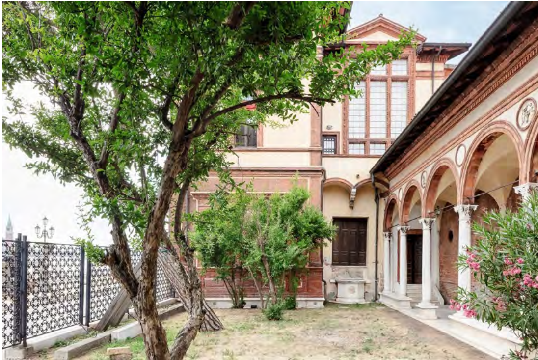
Figure 30 – View of Riva 7 Martiri historical headquarters of the Institute of Marine Sciences, where the equipment is installed.
