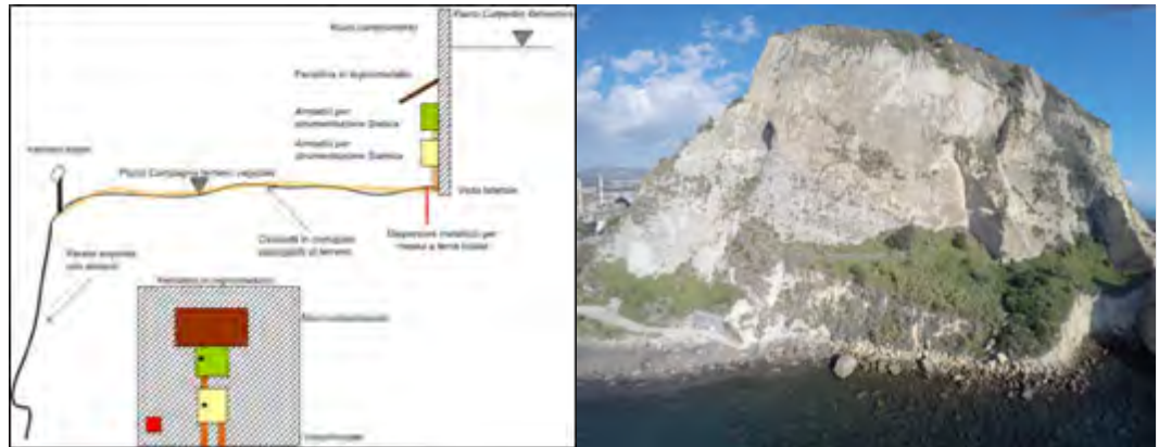
Figure 21 – MOSYS monitoring system of the Coroglio cliff (Naples).
