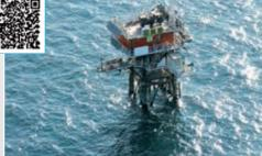
Originally installed in March 1970, after 46 years of scientific research activity, the Acqua Alta Oceanographic Tower is now undergoing a complete renovation program, which envisages a reinforcement of the underwater structures and a throughout refurbishment of the superior structures and technological systems, including the elevation of the main decks of about +2.00 m.
